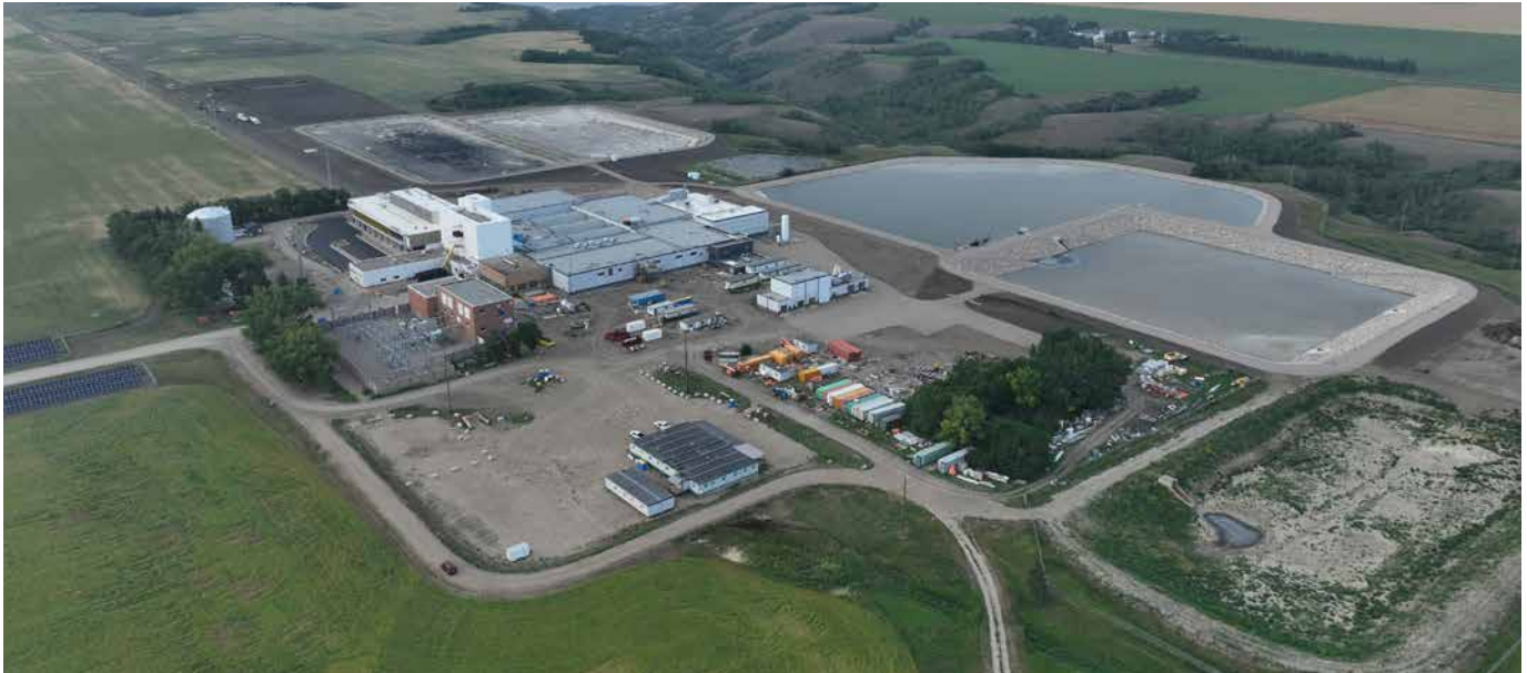
Figure 4: Construction of Summer Ponds A and B (right) were completed in 2023. Construction of Winter Pond A was completed in November 2024 (left centre) and a smaller than originally designed Winter Pond B (upper left) was completed in June 2025.
